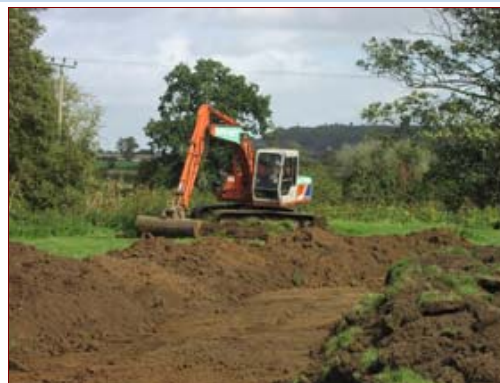
Photo 3. Creedy Bridge - Digger scraping the turf and topsoil in preparation for building the low retention banks along the Parrett. Ham Hill in far distance (14 Sept 2004) .
